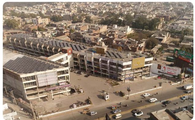
Prism Energy's first installation of 248 kWp on Pearl City Tower, in Faisalabad, Pakistan.
