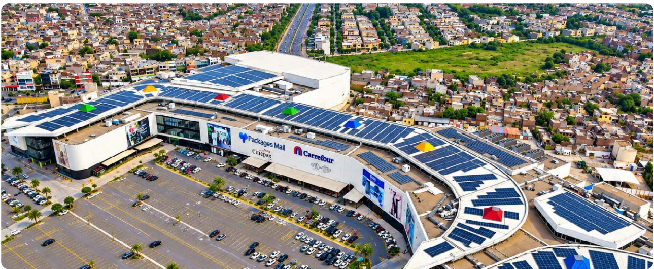
One of Shams Power’s largest installations on Packages Mall in Lahore, Pakistan. The image shows approximately 1.8MW of the 3.7MW rooftop installation.
