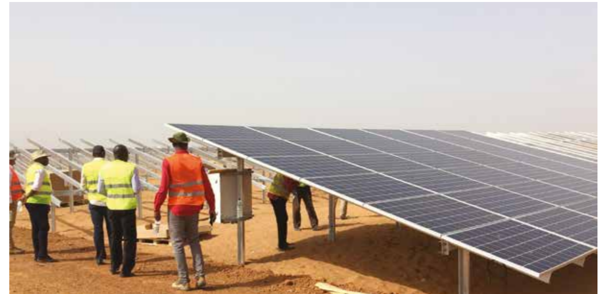
Senergy 2 solar park, Senegal
