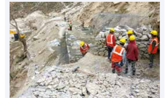
Construction workers begin work on the Lower Solu hydro plant
