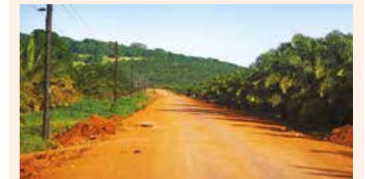
Bugala Island's newly-constructed Luuku to Mulabana main road.
