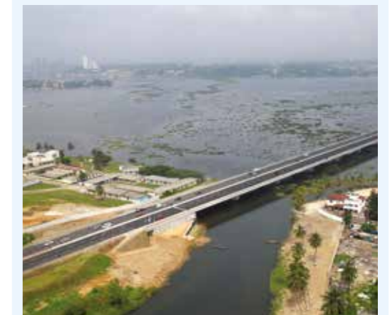
The HKB Bridge provides a vital new transport link for Abidjan
