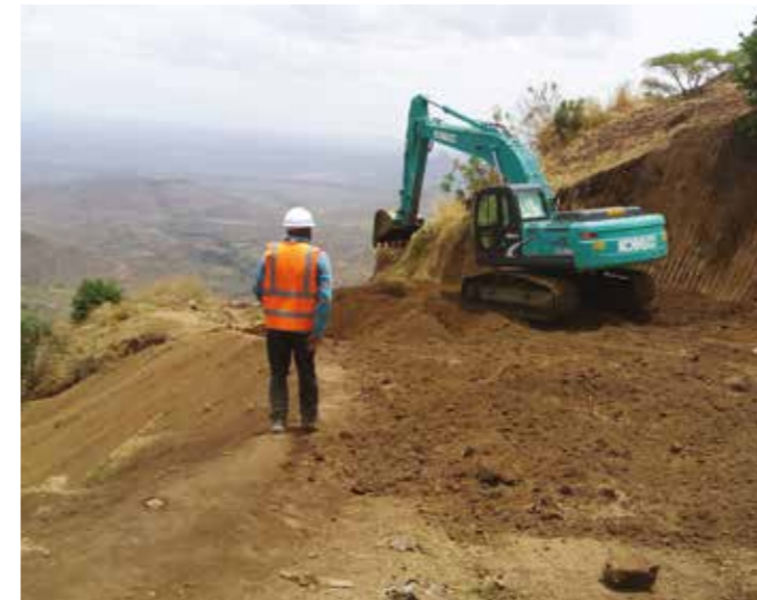
Work begins on road access to Siti II's power house
