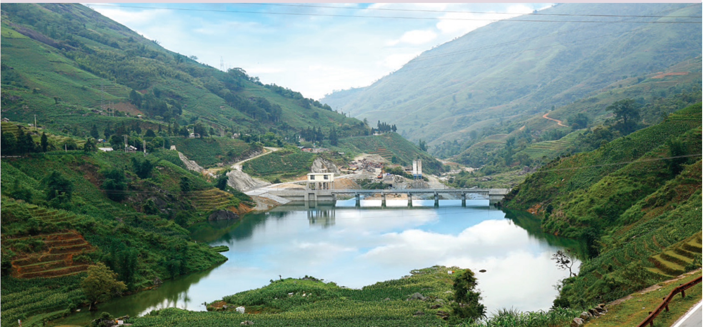
Coc San hydroelectric power plant | Lao Cai province, Vietnam | With Lao Cai Renewable Energy
